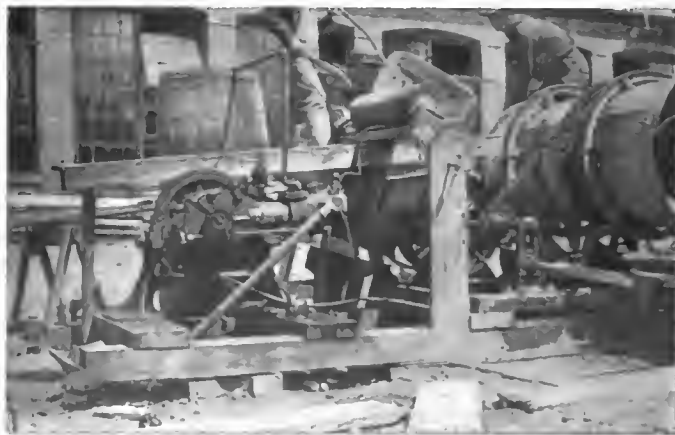
HOW THE OLD RAMBLER ENGINE TURNS THE CONCRETE MIXER.
